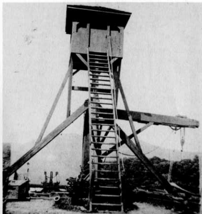
Fig. 11.13. Enlarged half of a Civil War era stereograph of the West Point Foundry cannon hoist tower, observation cupola, and gun hoist crane. Courtesy of the Putnam County Historical Society, Cold Spring.
