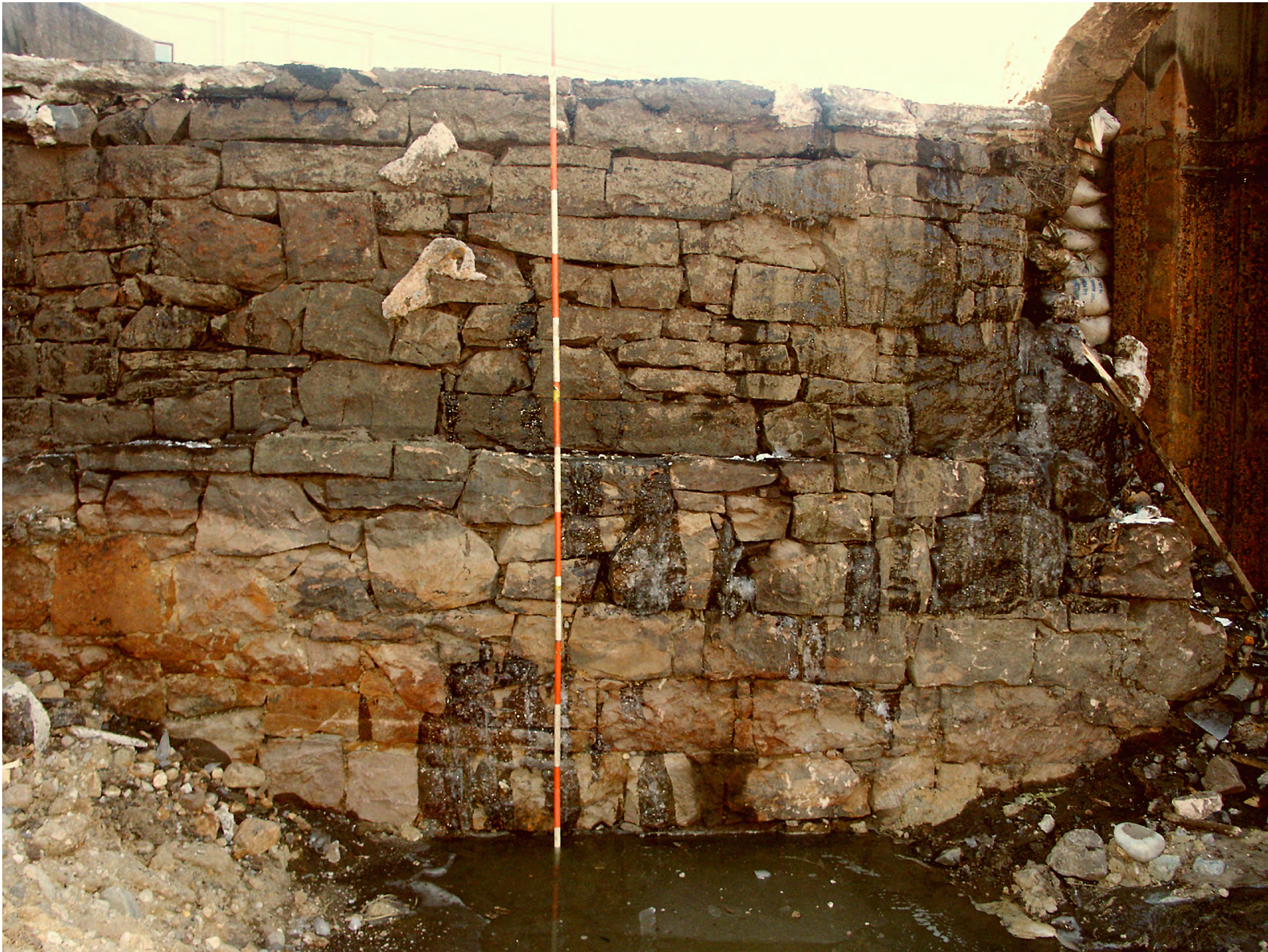
Figure 26: Digital macro photograph of east facade of Furnace Falls cut stone dam taken with natural light on afternoon of LIDAR scan, January 21, 2004. Note iron oxide stains and lighter band denoting depth of historic channel sediments.
