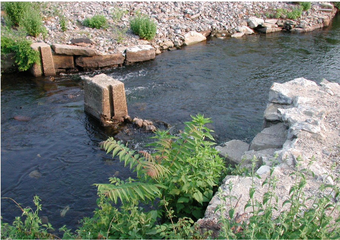
Figure 31. View looking, downstream, south-west across protruding and slotted post-1927 cement pods immediately upstream from former stone arched bridge (Photo by Joel W, Grossman, Ph.D.).
