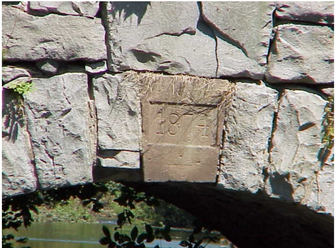
Figure 25. Detail of 1874 capstone in former cut stone arched bridge at Furnace Pond ( Photo courtesy of NJDEP )
