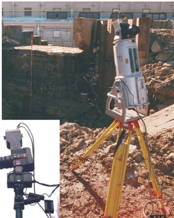
360° Riegl LIDAR Scanner & Rolleimetric Camera (Inset)
