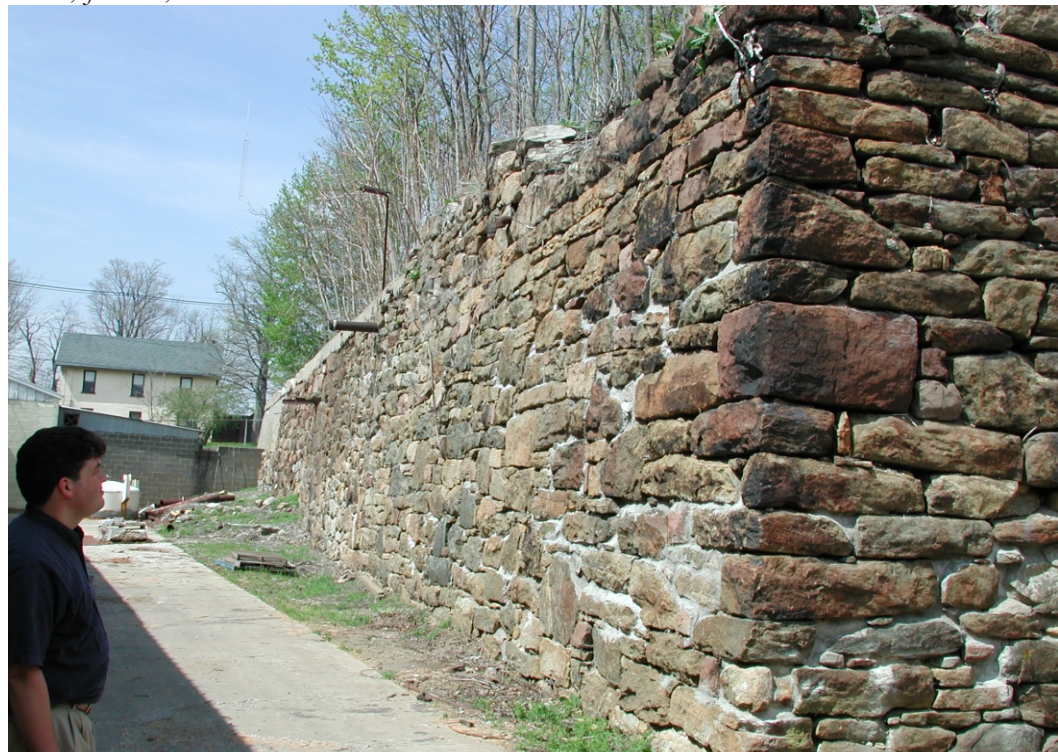
Figure 9. Modern view looking north along 16 ft. high, post-1840 stone retaining wall supporting interior blast furnaces and “L” shaped Morris Canal spur to the Foundry. Note fire reddened stones from former furnaces. (Photo By Joel W. Grossman, Ph.D., April 19, 2002).
