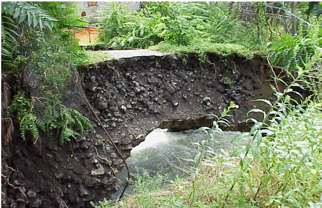
Figure 27. View looking south at deep scour channel through northern half of earth filled cut stone clad arched bridge at Furnace Pond ( Photo courtesy of NJDEP )
